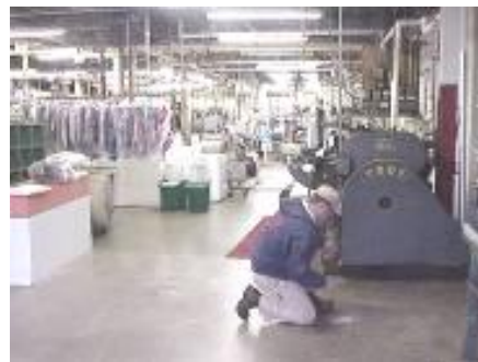
Note: Dry cleaner operations continue, no obstructions on surface after installation.
